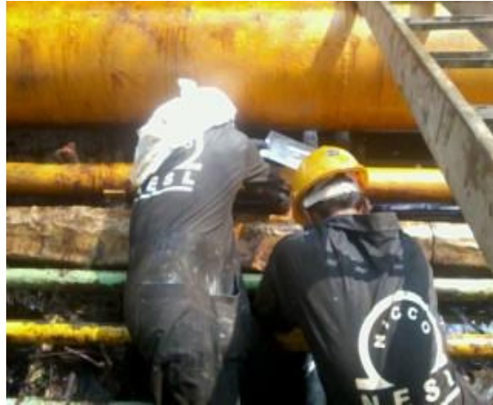
Repairing Job Under Process
