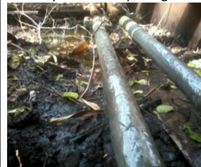
Pipes After Repairing
